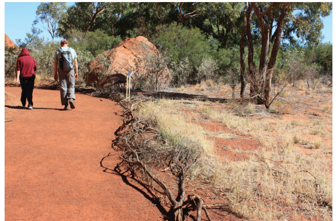
Good trail design can encompass re-use of material. At Uluru, the trail builder has used debris from trail clearing to prevent creation of unwanted paths.
