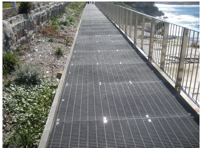
Fibreglass Reinforced Polyester (FRP) Mini-Mesh Grating is rapidly increasing in popularity as a walkway surface in sensitive reserves, such as here at Waverley in Sydney.
