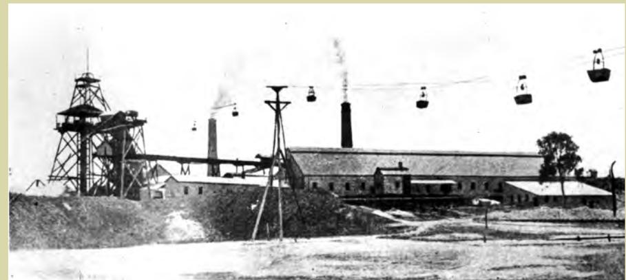
In 1911, a flying-fox (aerial tramway) was constructed to deliver ore from the No.3 shaft (unseen on right) to the crushing battery adjacent to the No.1 shaft.
