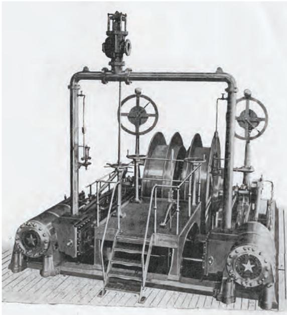
A steam winding engine manufactured by Walkers Ltd for the Oriental Consols Gold Mining Company in 1900. This plant consisted of a pair of coupled twenty inch cylinders with forty-two inch stroke and a pair of eight foot drums with a one inch rope 2,750 feet in length. The Cornish boiler was twenty-seven feet long and seven feet in diameter. Source: The Gympie Times, 1910.
