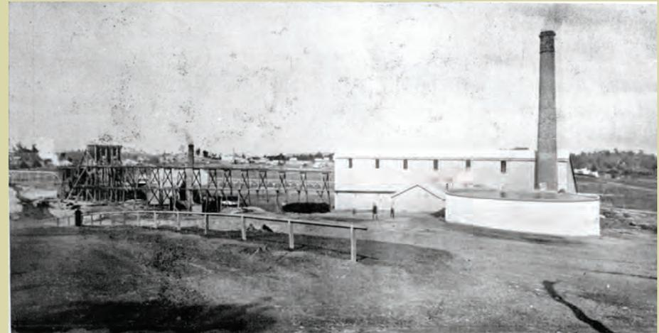
Mine buildings including tramway, battery and concrete water tank at the eastern shaft of the 2 South Great Eastern in 1903. Today the tank is part of the display area of the museum. Source: The Gympie Times, 1903.
