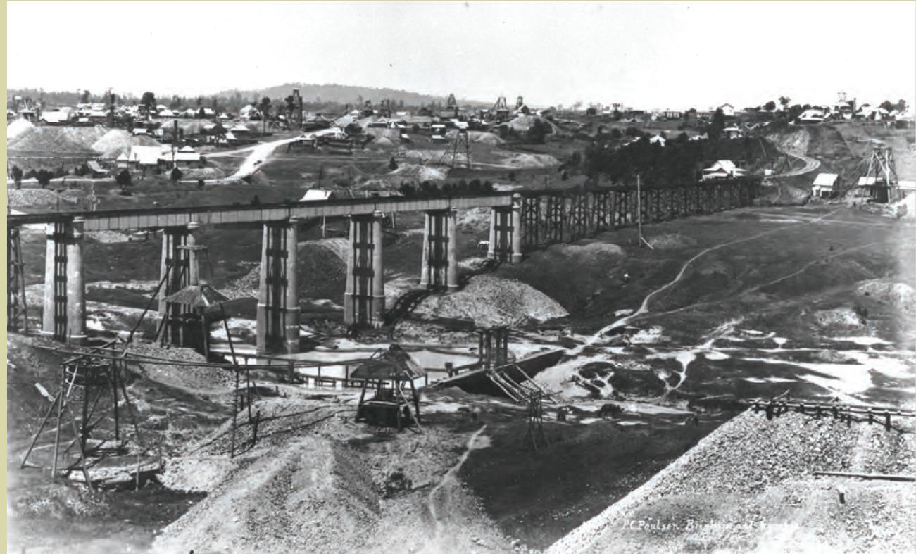
The Deep Creek bridge on the Brisbane rail line, circa 1899. Note mullock, old shallow shafts and weir in the foreground and numerous headframes at Monkland in background. On the left above rail bridge is the Victoria battery. Photographer: P. Poulsen. Source: Lees, W. 1899.
