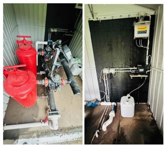
Figure 4-3. Filtration and chlorine dosing on the drinking water plant
