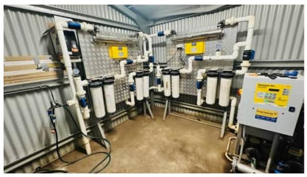
Figure 4-1. Overview of filtration and UV disinfection
