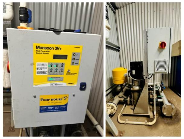
Figure 4-2. Variable speed pump controllers, pumps and pressure vessel
