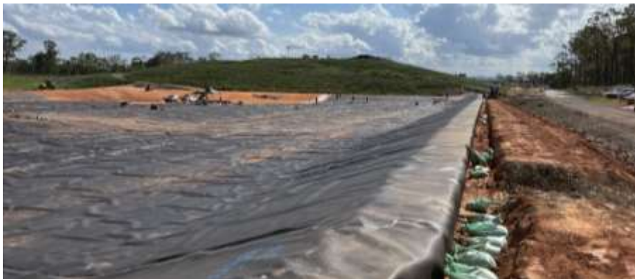
Eastern Cell construction & black liner
