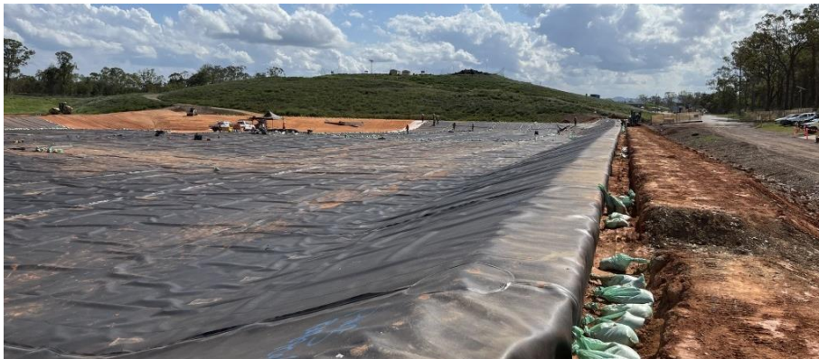
Eastern Cell construction & black liner
