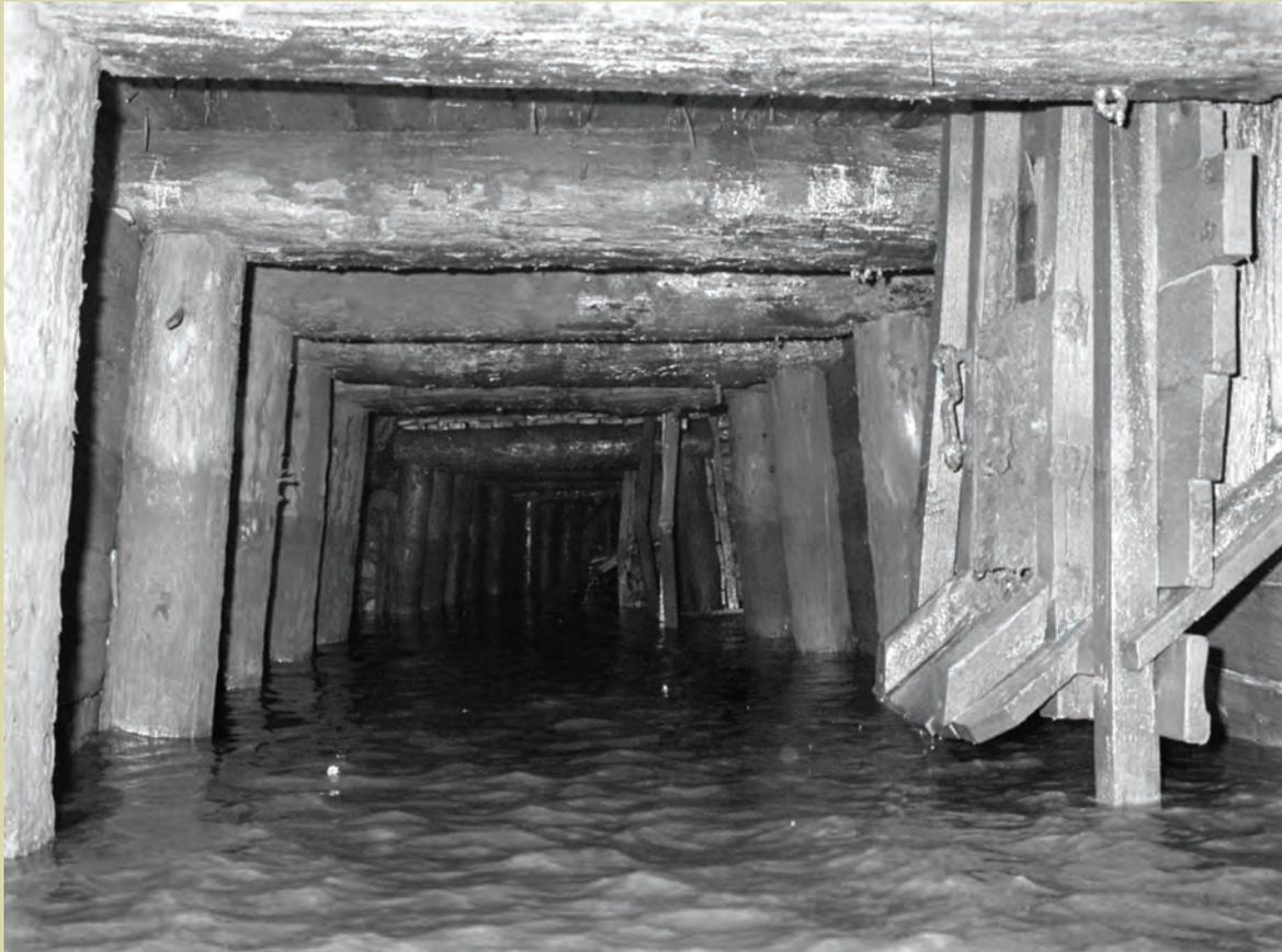
Old timber structures below the Scottish No.3 shaft, exposed after the dewatering of the old workings through the West of Scotland shaft. Photographer: Bernie Crawford. Source: The Gympie Times, 1990.
