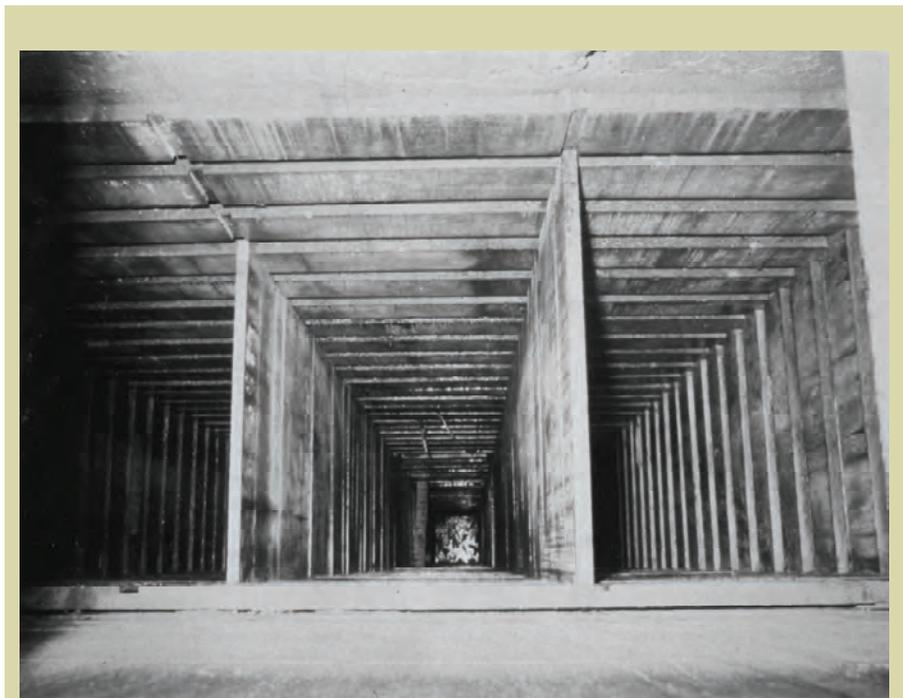
Looking down the exposed three chambered timber lined shaft of the West of Scotland, November 1986. Note the water at the bottom.
