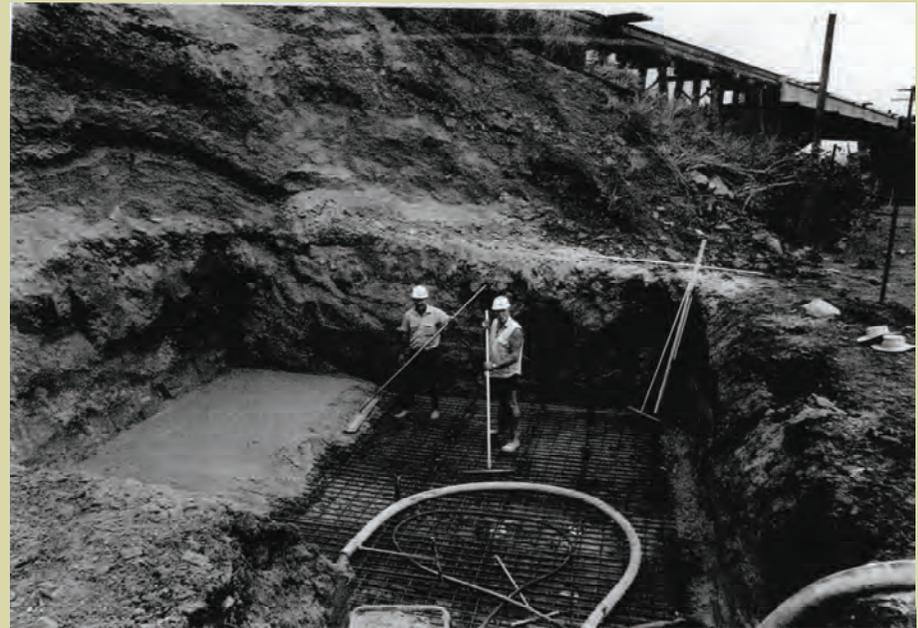
The Shaft Capping Project team places a concrete cap over an exposed mineshaft.
