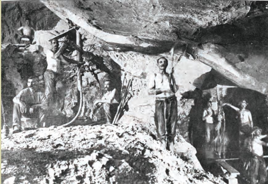
Miners at work in the East Oriental and Glanmire mine in 1910. Note the two rock drills, the flat reef and the hot working conditions.
