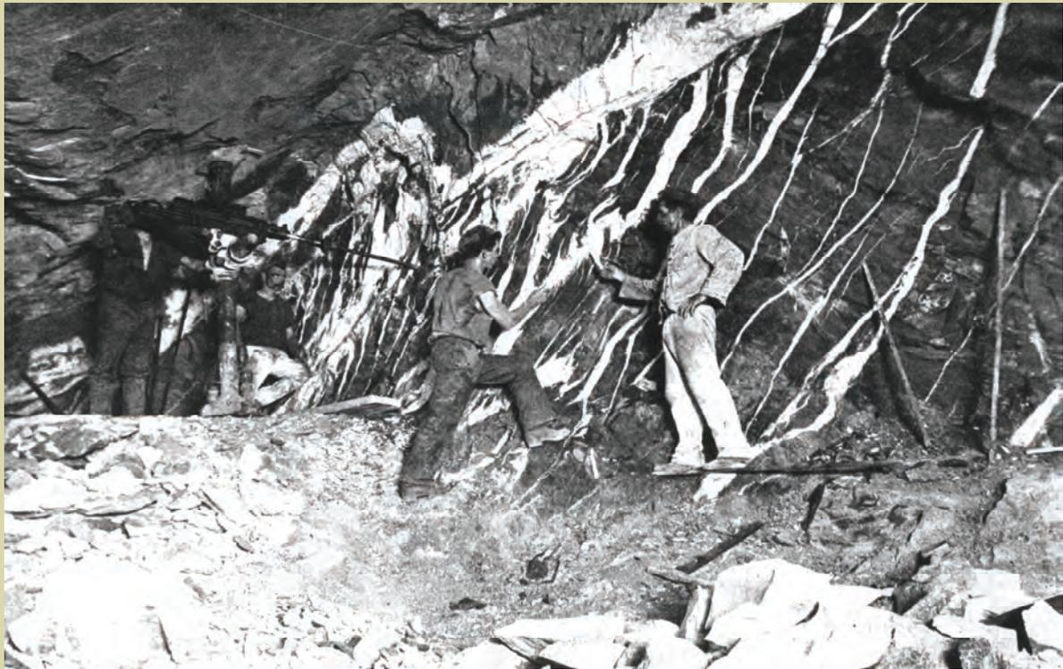
Miners at work on the No.2 reef above 1,282 ft, level at the 2 South Great Eastern, 1902. Note the drill on left and mine manager Jack Harris on right.
