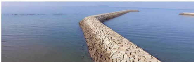
Breakwaters are erosion control structures most frequently placed parallel to the coast. Breakwaters are typically constructed using rock or geo-bags. **Exposed breakwaters** have a crest that rises above the surface of the water, whereas **submerged breakwaters** do not.
